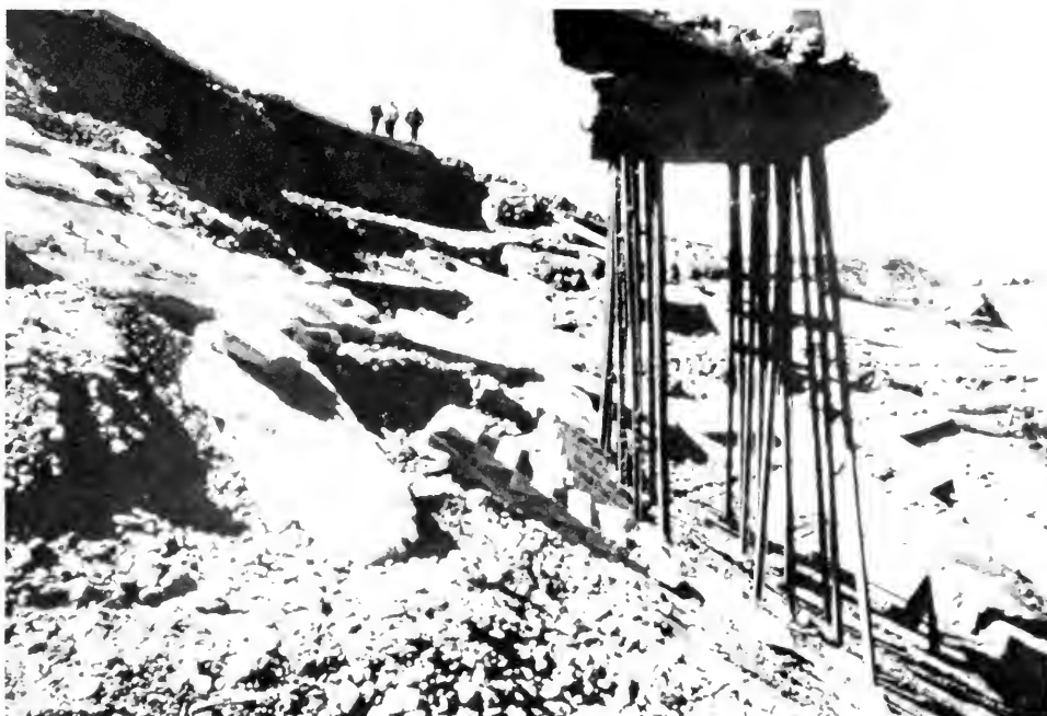
Photo 3. Pile-supported footing for foot bridge to intake tower after slide.
